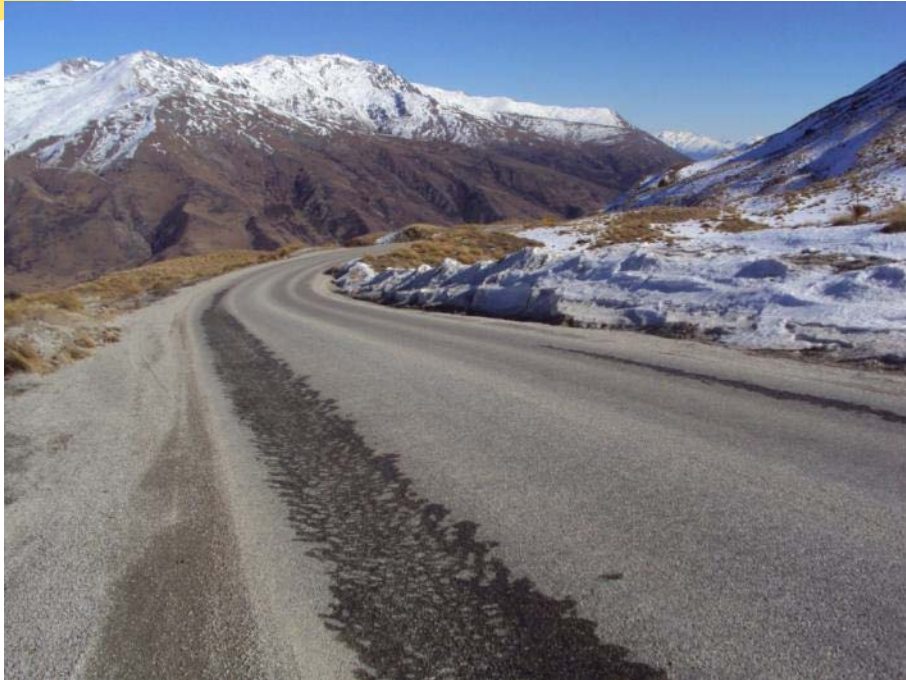
Ongoing Crown Range Road Rehabilitation and many other rural arterial sites.
