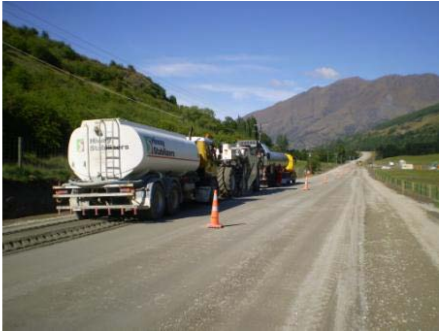
Malaghans Road Site 1 Rehabilitation and Widening 2009-10.
