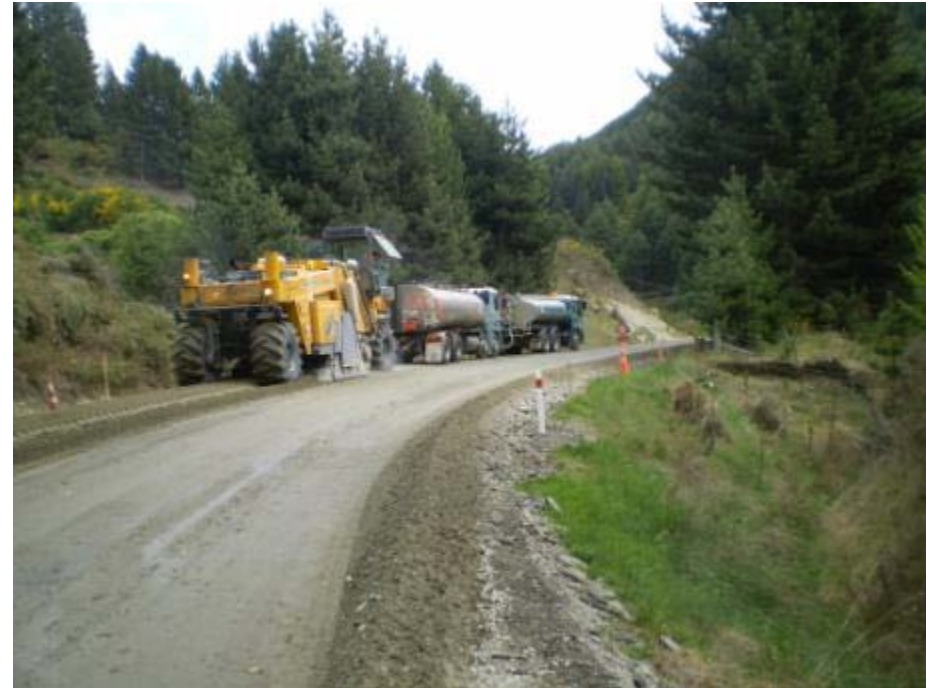
Glenorchy Road Pavement Rehabilitations 2009-10
